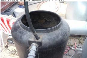
**Photo A.4.** Holding tank, (collection reservoir for the UASBs' effluent). The photo shows also the overflow line from which excess pretreated sewage is conveyed back to the grit chamber.
