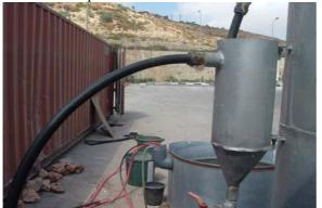
**Photo A.3.** Connecting container which collect the UASB-septic tank effluent. The photo shows also the hose which convey the effluent to the holding tank (see photo A.4).
