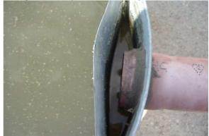
**Photo A.6.** The baffle which was installed for preventing short circuiting of wastewater and to prevent floating materials from transporting to successive stabilization ponds. The 4" PVC pipe connecting stabilization ponds is also shown
