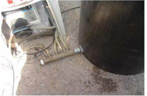
**Photo A.5.** Suction point from the holding tank by the pumps to the stabilization ponds. The MASTER FLEX hoses are also shown. The photo shows also the pump feeding the deepest stabilization ponds.
